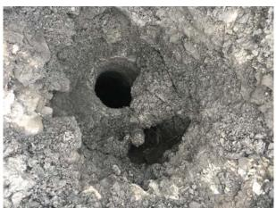
The procedure for locating and mapping out blasting patterns should include controls to prevent misalignment or overlap of patterns with previously shot ground. Additionally, blasting procedures should include inspections to identify misfired holes and the logging and communication to all relevant workers the location of these misfires.
