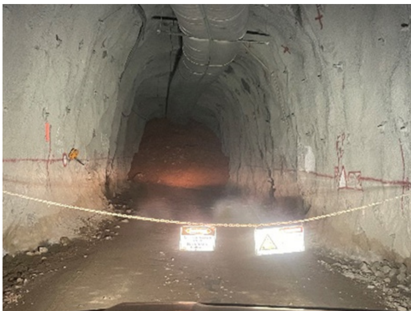
Picture 4. Liquified clay following the blast.
