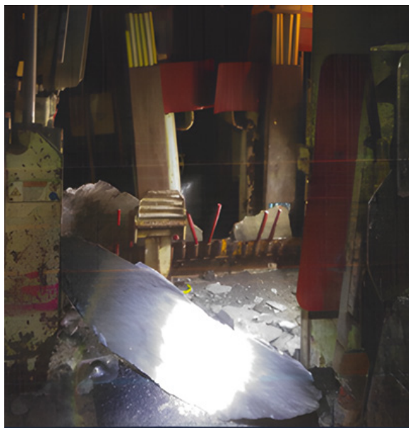
Picture 3. Large piece of stone fallen from roof.
