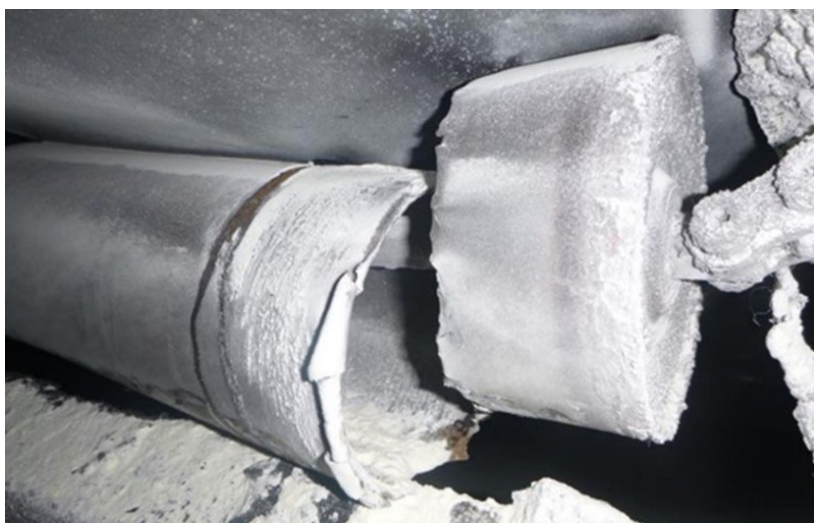
Picture 11. Fire damage.
