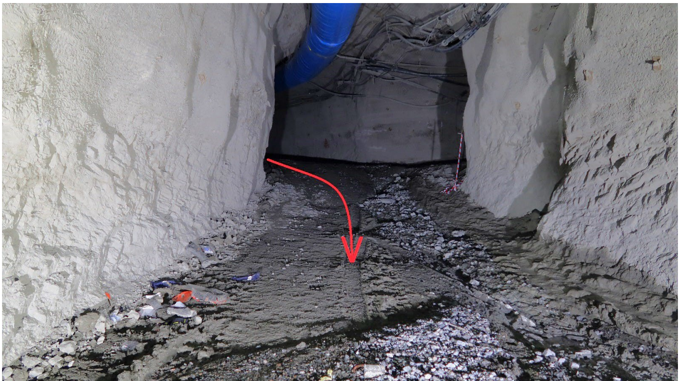
Figure 2: View of the point of collision facing up the decline with a red arrow indicating the loader's path of travel
