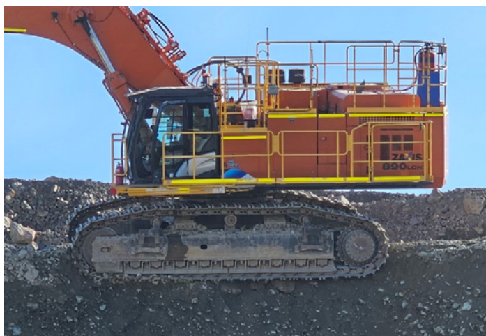
Picture 8: Excavator tilted on failed embankment.
