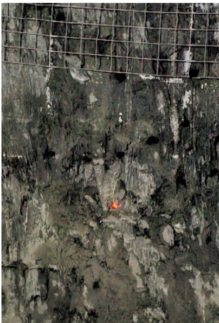
Picture 13. Flame in drill hole.
