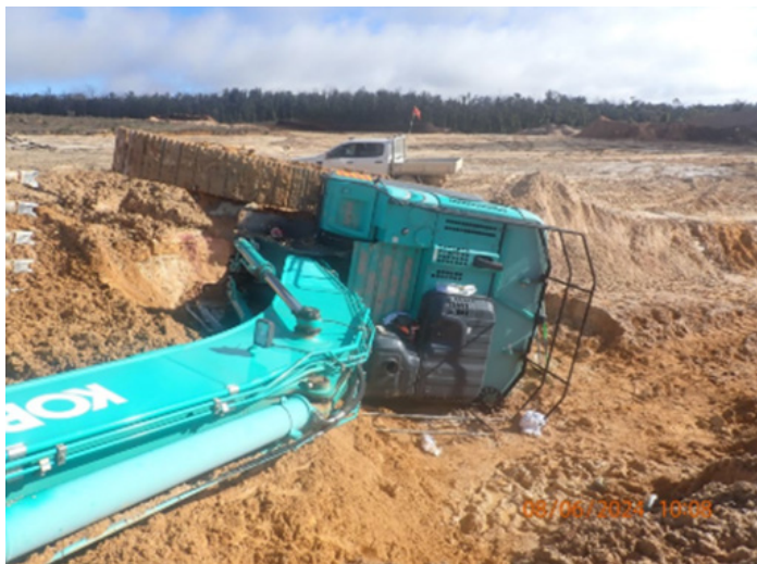
Picture 10: Excavator on its side.
