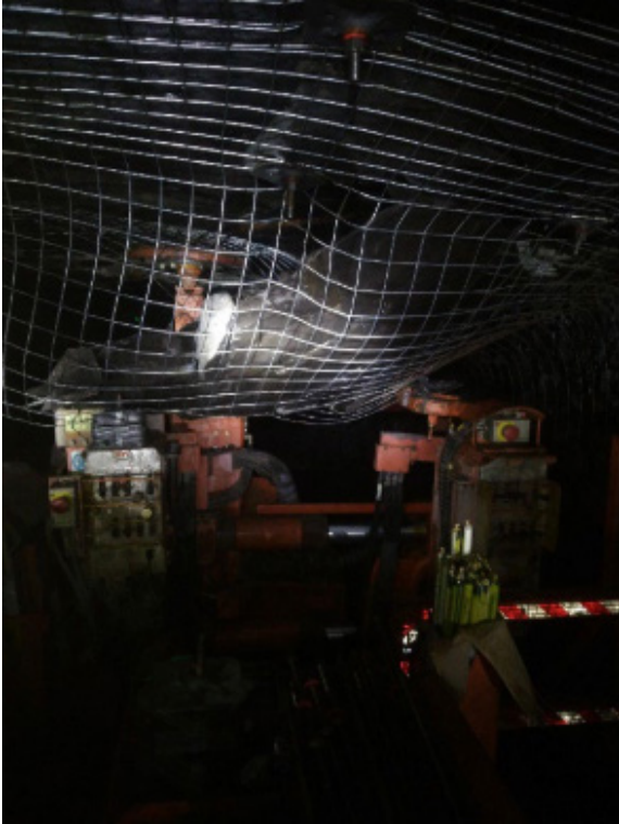
Picture 4. Material on mesh and timber jacks.
