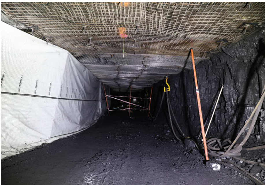
Figure 4 Photo outbye of the incident site
