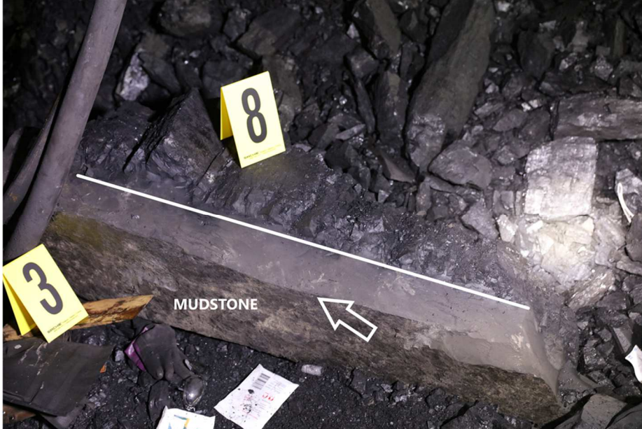
Figure 3 The coal and mudstone block (marked with No.8 'A' frame) which struck worker A
