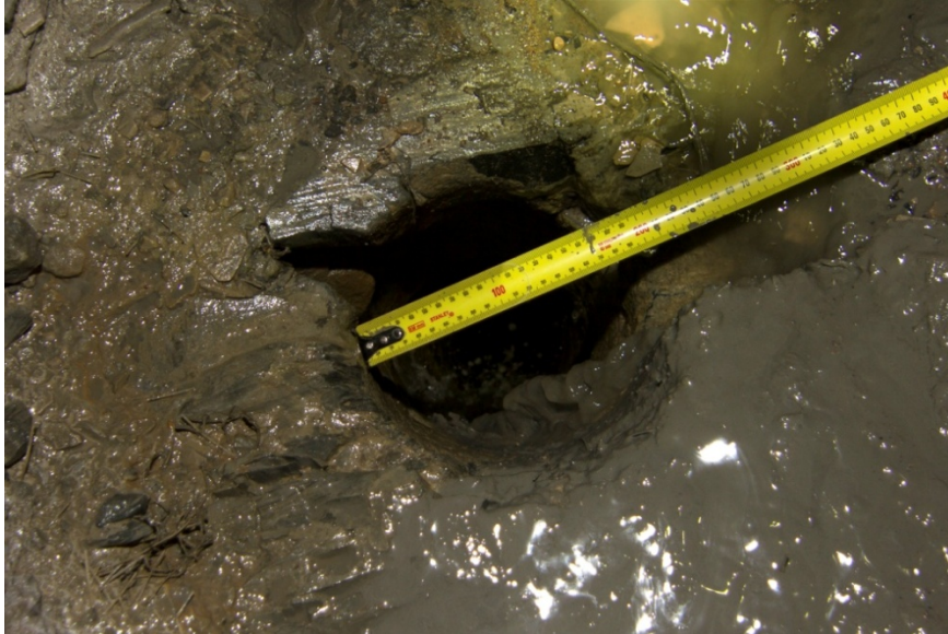
Borehole in the bottom of the incident sump - Photograph by Investigation Unit
