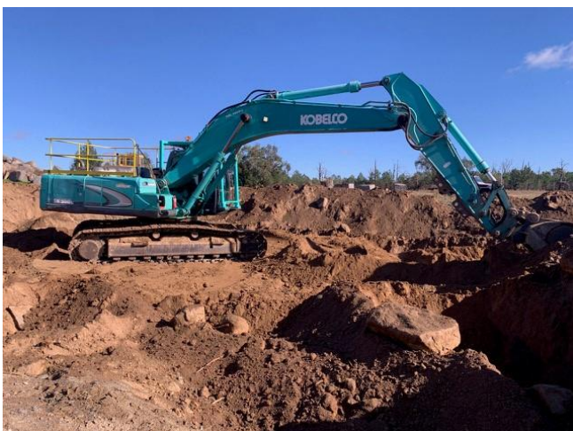
Figure 1 Excavator on site
