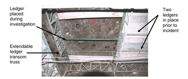
The ledgers (used as spreader bars) hold adjacent extendable transom trusses together to prevent sideways movement of the transom trusses.
