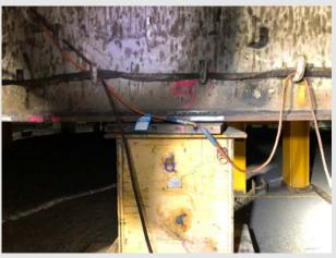
Welding machines must be isolated when not in use. Workers who are given tasks to clean work areas must be given clear instructions and must confirm that equipment is isolated before commencing work.
