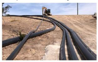
When poly pipe is being moved, the stored energy and potential for sudden release (spring back) must be taken into account in task procedures. Clear and defined 'no-go' zones must be developed to protect workers from sudden releases of energy.
