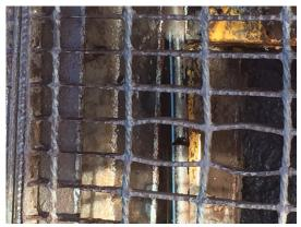
A job safety analysis (JSA) was completed for this task but did not identify the risk of the lines underneath the mesh floor being compromised. The pressure cleaner operating pressure was reduced for the job from a maximum pressure of 2500bar to 690bar.
