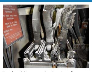
An electrician was going to a transformer following an overload trip on a supply circuit breaker to a DCB in a development panel when he smelled smoke.
