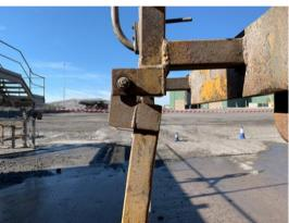
Mine operators should review their procedures to determine if their training includes the hazards associated with potential pinch points and their identification.
